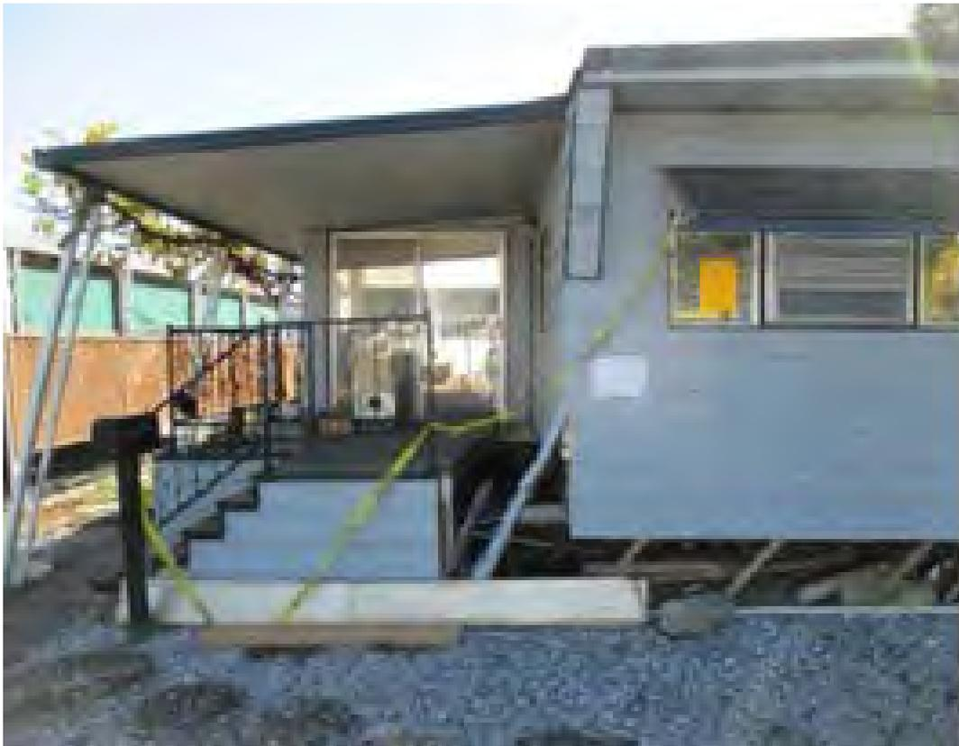
**Figure 1. Damage to Manufactured Housing Unit following the 2014 Napa California Earthquake Likely Due to an Inadequate Support System**
