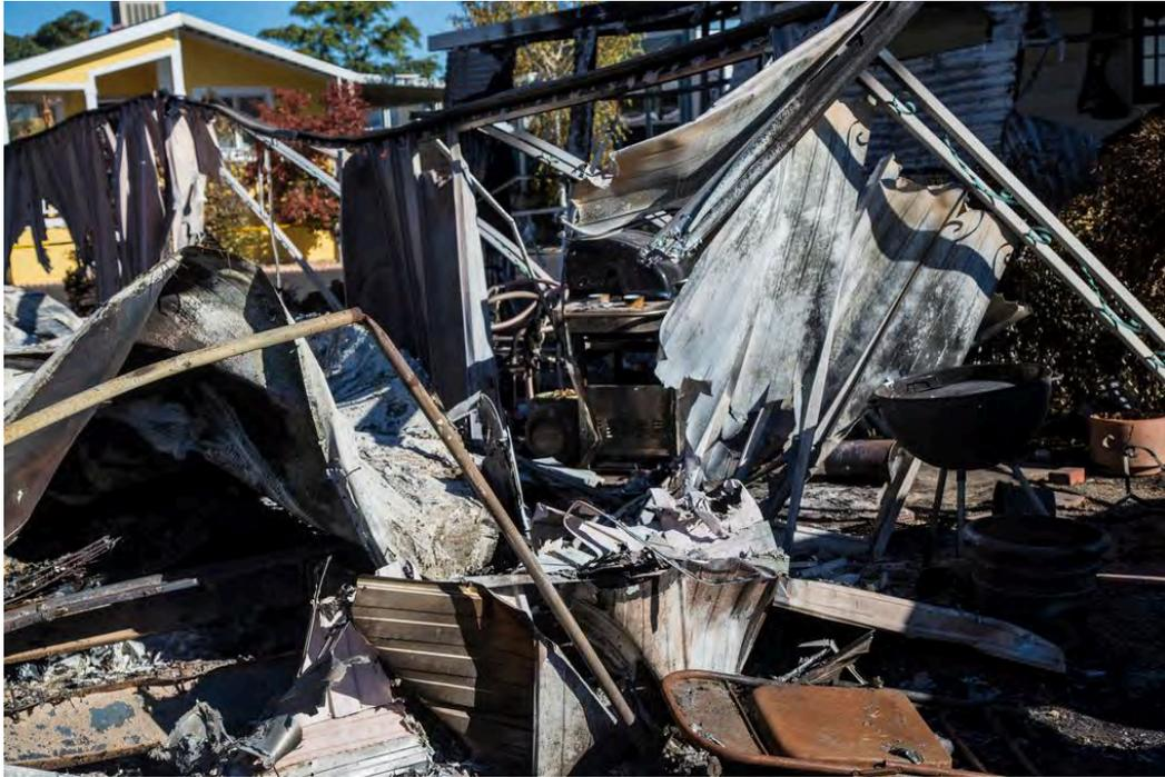
**Figure 2. Fire damage from broken gas lines at the Napa Valley Mobile Home Park which was struck by a 6.0 earthquake on August 24, 2014**
